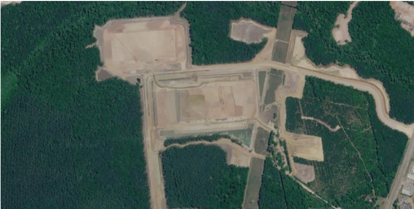
Port Wentworth Commerce Center, site work underway. Buildings A and B, a combined 1.28 million square feet, expected delivery Q4 2026, with Class I CSX rail on site. This aerial shows a portion of the site only and is not the full extent of the property, which is master planned to 10 million square feet across 18 buildings.
