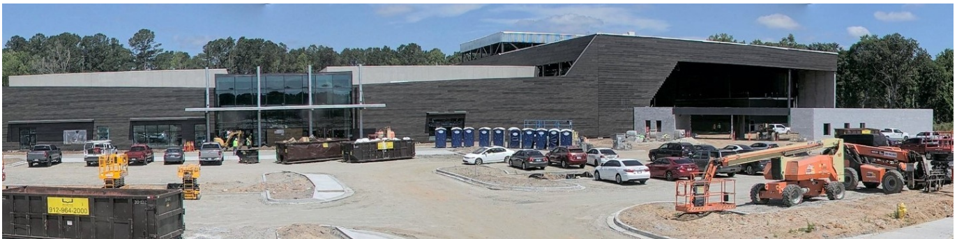
Anchor Park under construction, May 2026.
