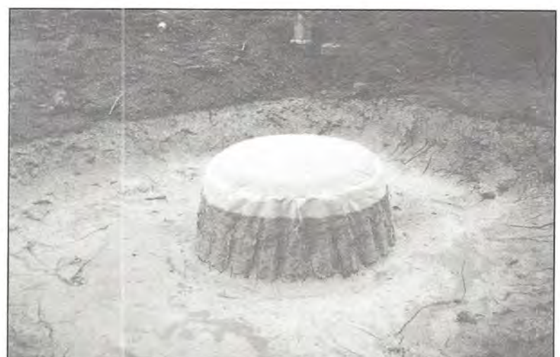
Figure 6-28.7 Equivalent Inlet Sediment Trap
