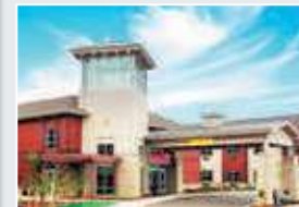
Lafayette Transitional Care Transitional Rehabilitation Center Lafayette, CO | 60,000 SF
