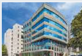
First Hill Medical Pavilion Acquired Outpatient Center Seattle, WA | 227,682 SF
