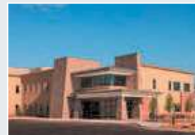
St. Anthony North Hospital (Centura Health) On-Campus Outpatient Center/FSED Westminster, CO | 48,000 SF
